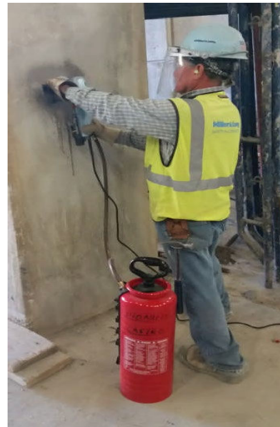
Example of a handheld grinder with integrated water delivery system.
