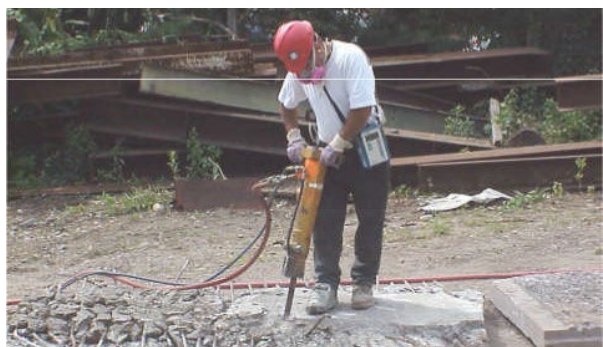
A worker chips concrete with a jackhammer using a water-spray attachment to control dust.
