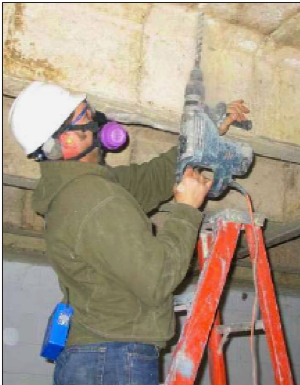
Rotary hammers can produce high levels of silica dust, especially when used directly overhead. (Photo courtesy of New Jersey Department of Health and Senior Services, Silica Surveillance Project).
