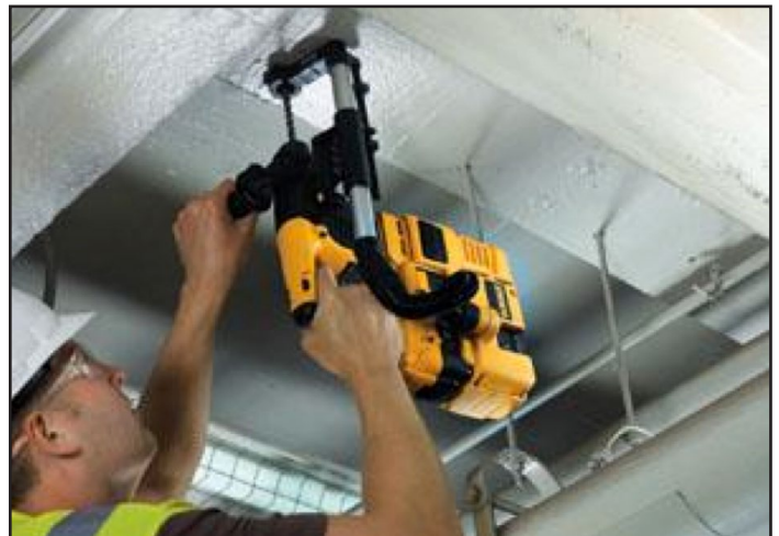
Rotary hammer with built-in VDCS including HEPA filter. Note the shroud, hose and vacuum. (Photo courtesy of DeWalt. The equipment shown in this picture is for illustrative purposes only and is not intended as an endorsement by OSHA of this company, its products or services).
