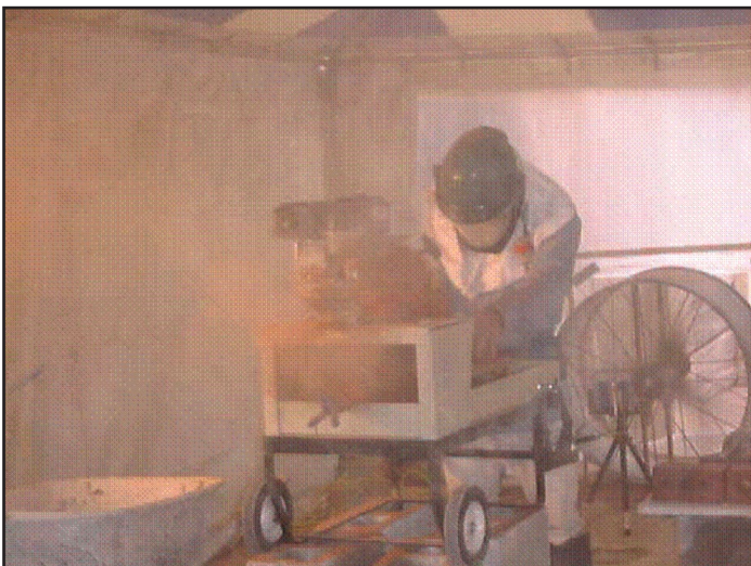
Stationary saws operated with no dust controls create large amounts of silica dust. (Photo courtesy of the University of Washington).
